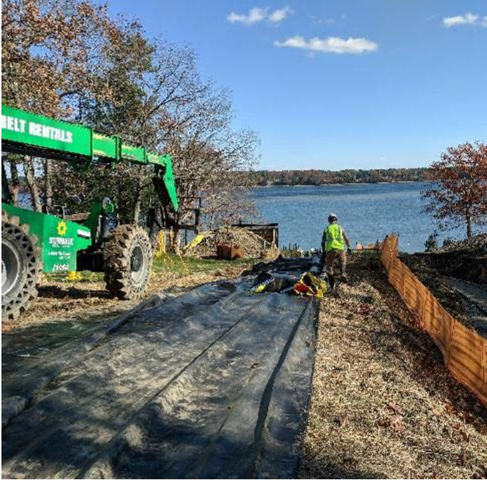
Fig 25: Deploying the turbidity barrier for hand jetting at the Getchell property Viewing east. (11-06-19).
