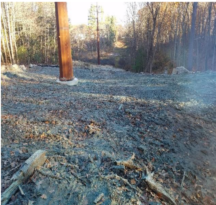
Fig 11: Hydro-seeded area around Str. 29. Viewing north. (11-02-19).
