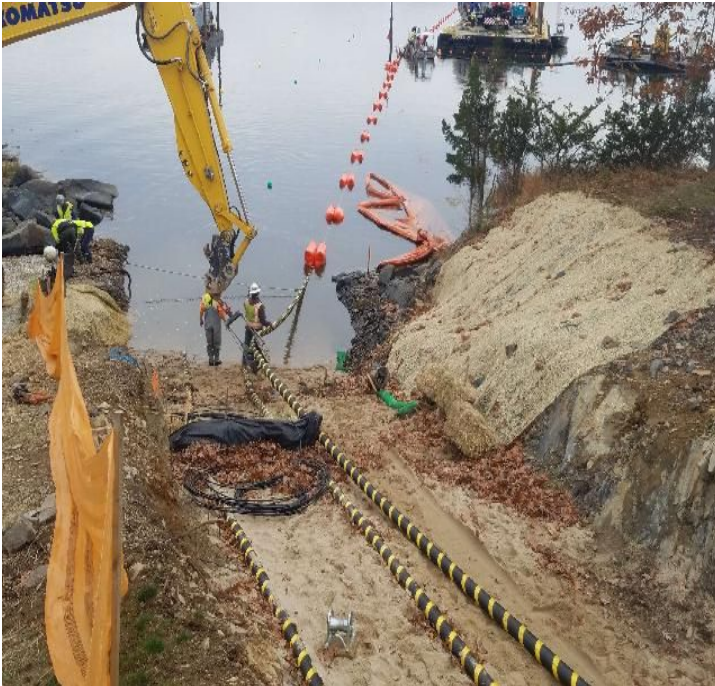
Fig 21: Landing cable at Getchell property/west side of the Bay Viewing east. (11-05-19).
