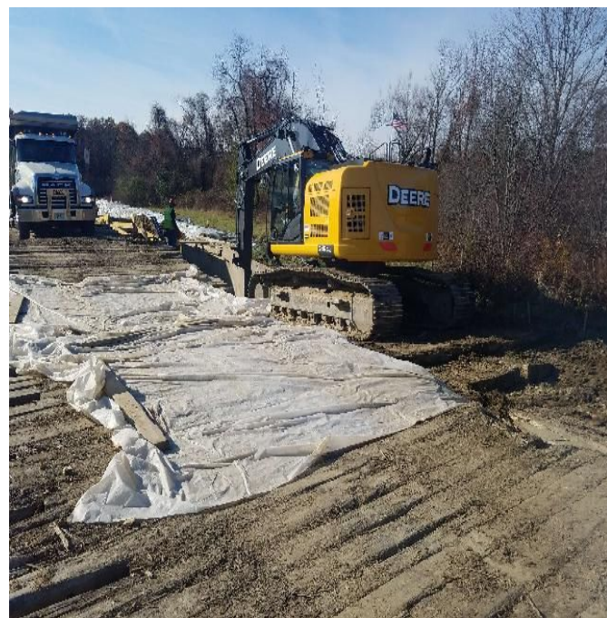
Fig 16: Beginning to trench through wetland NW18 at Frink farm. Viewing east. (11-04-19).
