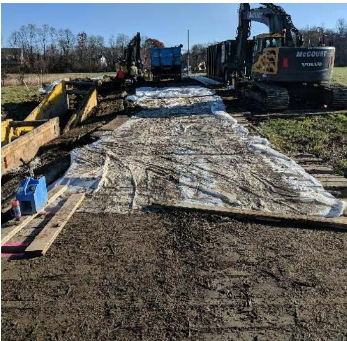
Fig 23: Poly sheeting over timber mats at Frink farm. Viewing east. (11-06-19).
