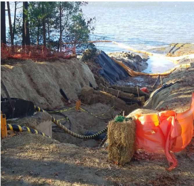
Fig 3: Triple row of sediment controls in trench at Gundalow Landing/east side of the Bay. Viewing west. (11-01-19).
