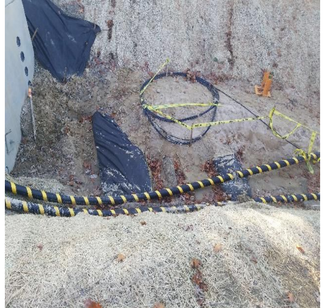
Fig 14: Sediment controls in trench at Gundalow landing/east side of the Bay. Viewing south. (11-04-19).
