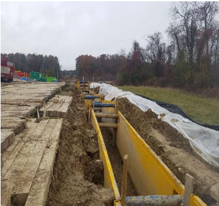
Fig 19: Trenching through agricultural zone at Frink farm. Viewing east. (11-05-19).
