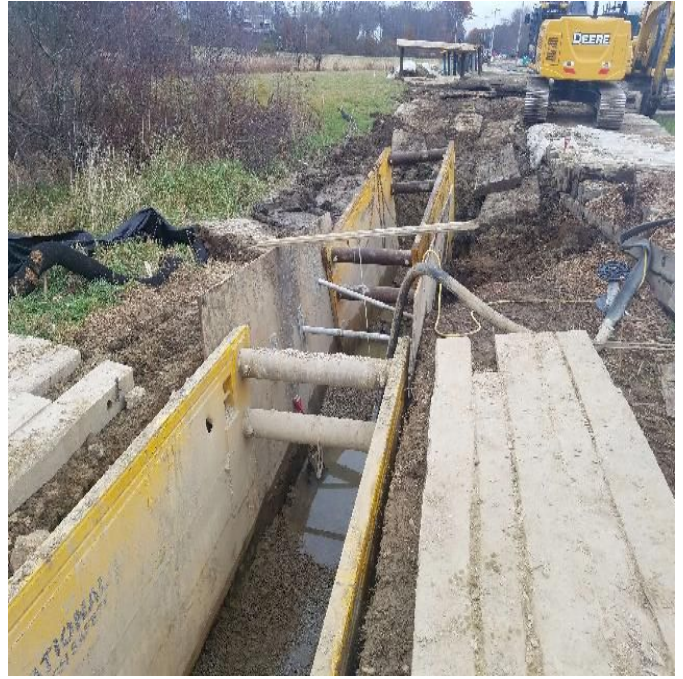
Fig 18: Pumping groundwater out of trench in wetland NW18. Viewing west. (11-05-19).
