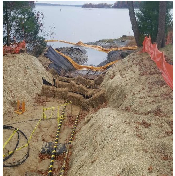
Fig 22: Sediment controls in trench at Gundalow landing/east side of the Bay. Viewing west. (11-05-19).
