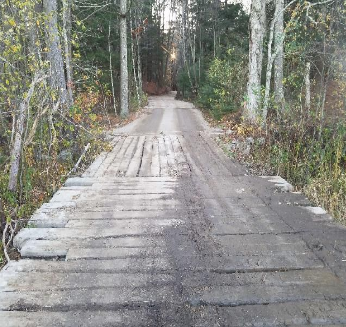
Fig 9: Access road to Str. 9-13. Viewing east. (11-02-19).
