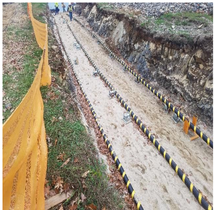
Fig 20: All three cables landed on shore at Getchell property/west side of the Bay. Viewing east. (11-05-19).
