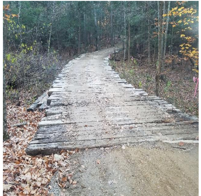
Fig 10: Access road to Str. 9-13. Viewing east. (11-02-19).
