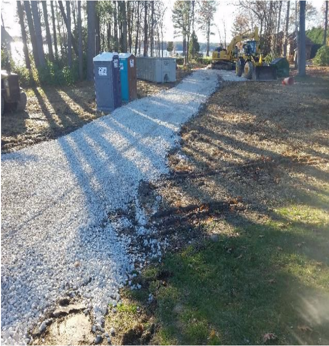
Fig 5: Crew placed fabric and stone on access to trench at Gundalow Landing/east side of the Bay. Viewing west. (11-01-19).
